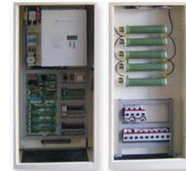
Control Panel (For Lift Passenger, Service, Cargo, etc) Type:CMH01
